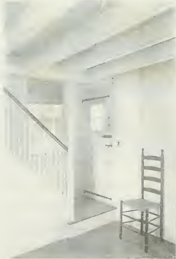
Figure 42 Stair and Rear Entrance, First Floor of North Wing, c. 1930
